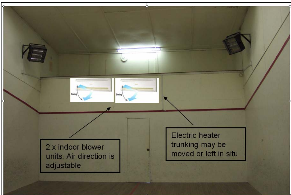
FIGURE 1a - Estimation of how inside blowers will look. Offset in this impression as we are not sure about moving the trunking (arrowed). No impression of protective grille available.
