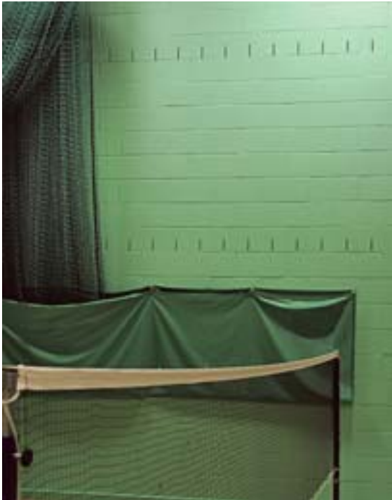
Figure 7 Note acoustic blocks have been used in the wall construction
