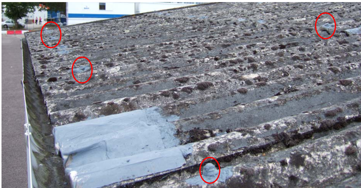
Enlarged view of all coated sheet cappings (circled as examples).
